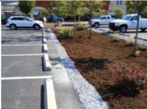
Gravel diaphragm – flow enters as sheetflow and is evenly distributed across length of practice
