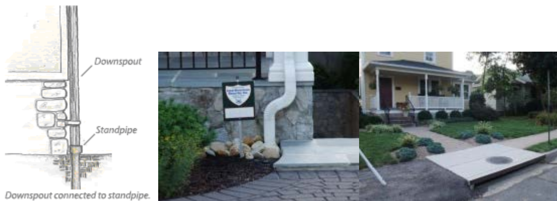
Figure 1: Different ways a downspout can be connected. Starting at the left: Downspout connected to sewer intake pipe (standpipe), downspout directly connected the storm sewer system, and downspout discharging to driveway, which discharges to road and storm sewer system.
